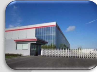
Jinshan, Shanghai Pressure vessel 120,000 m2
