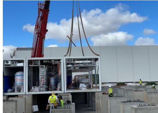
Module lifting
