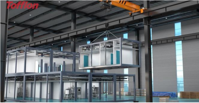
Steel frame fabricate
